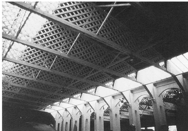
Figure 13 Belfast roof truss for an aircraft hangar at Duxford, England.
