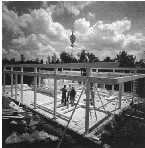
Figure 19 Completed assembly of the ground floor.
