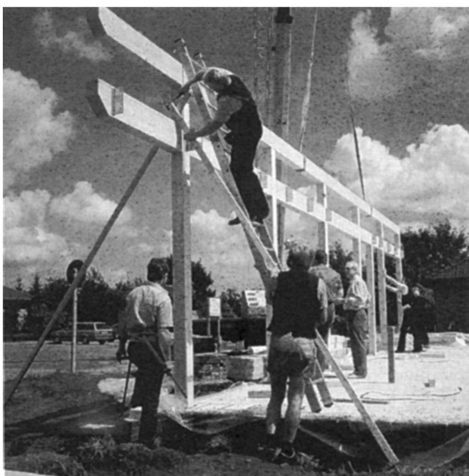
Figure 16 Assembly, alignment and fixing of the first structure in one axis.
