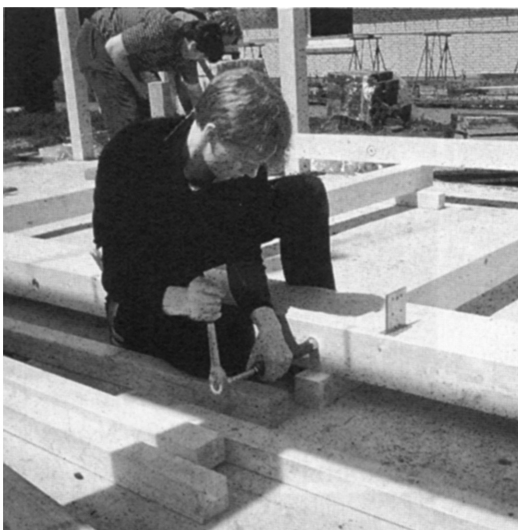
Figure 15 Assembly of columns and main supporting beam.
