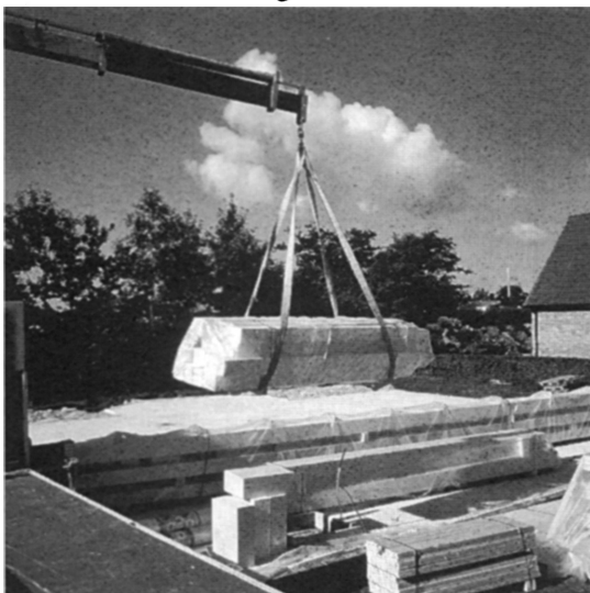
Figure 14 Delivery of complete beam and post structure components to the building site.
