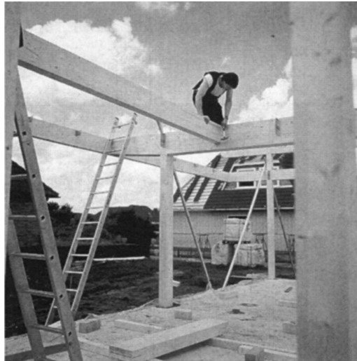
Figure 18 Placing of the secondary beams.
