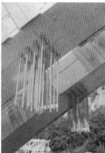
Figure 41 Detail of connection between hanger and arch.
