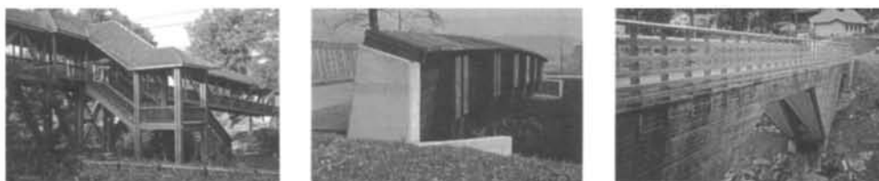
Figure 8 Effective protection against the influence of the weather: (a) traditional roof, (b) easy to replace inclined and vertical cladding, (c) waterproof deck with lateral cladding.
