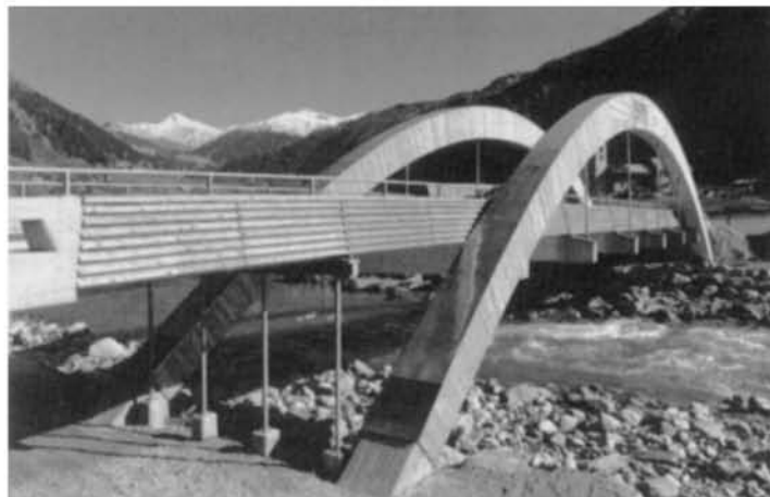
Figure 38 View of the glulam arches of the San Nicla bridge.
