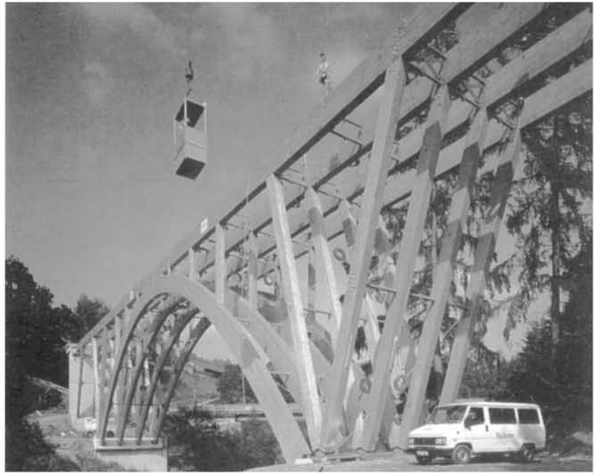
Figure 34 Deck seen from below with three-hinged arches, longitudinal beams, inclined columns, columns on arches and bracing.
