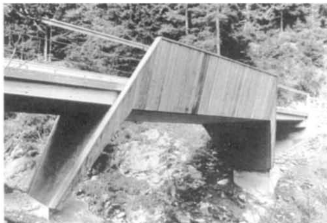
Figure 25 View of the cladded strut frame.
