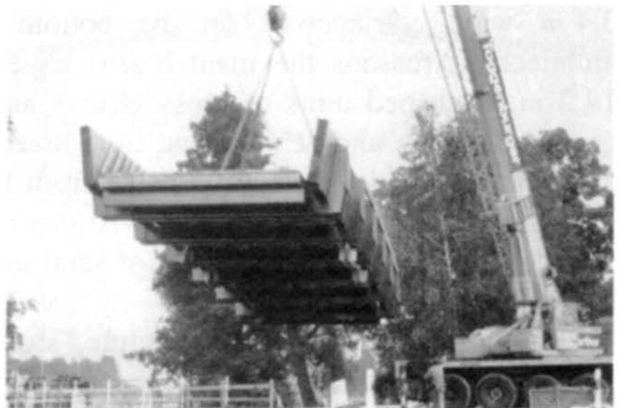
Figure 22 A mobile crane is used to erect the bridge.
