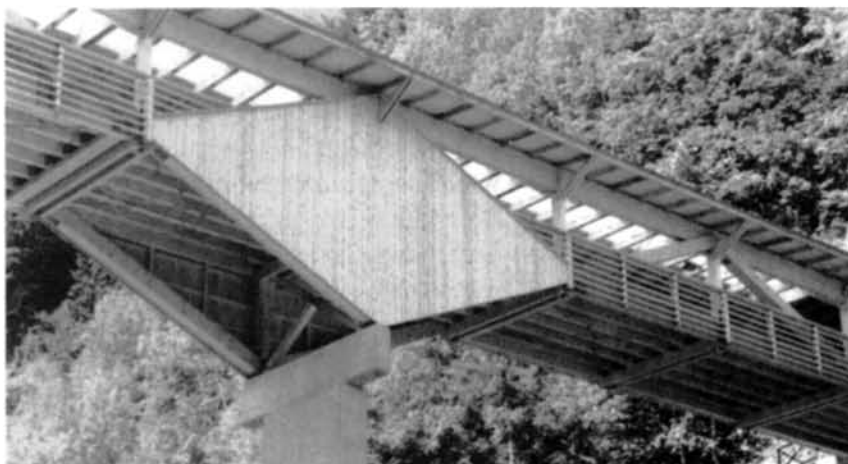
Figure 20 The transparent looking bridge rests on concrete piers.
