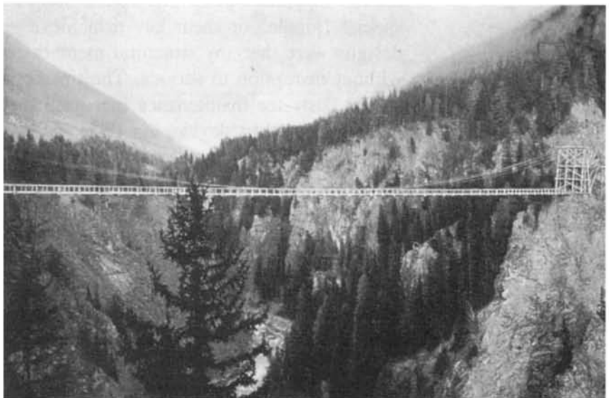
Figure 5 Suspended bridge close to Brail (1910) used for material transports to a tunnelling building site; span 168 m, 60 m above the river Inn.
