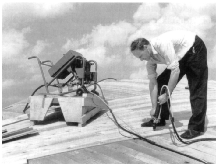
Figure 13 Fastening of the membrane layers.
