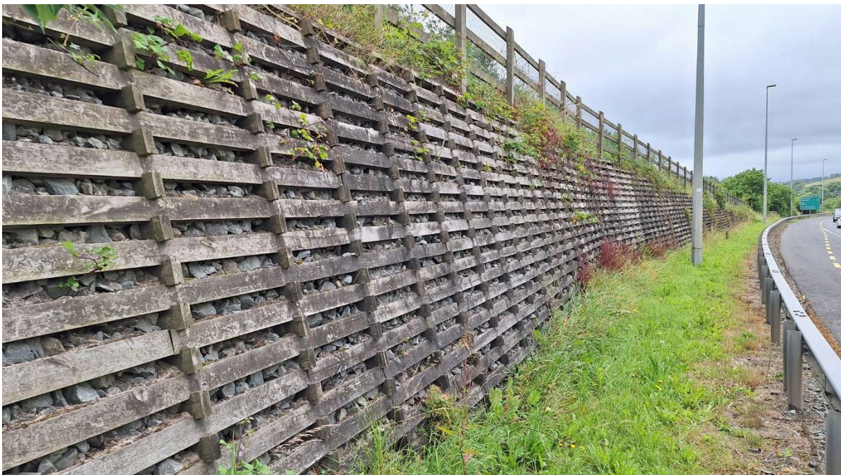
Figure 6: Crib retaining wall beside a national roadway
