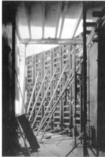
Figure 6 Frame-type formwork system.
