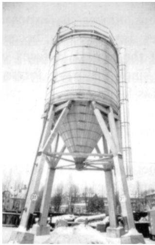
Figure 2 Silo from glulam for salt storage.
