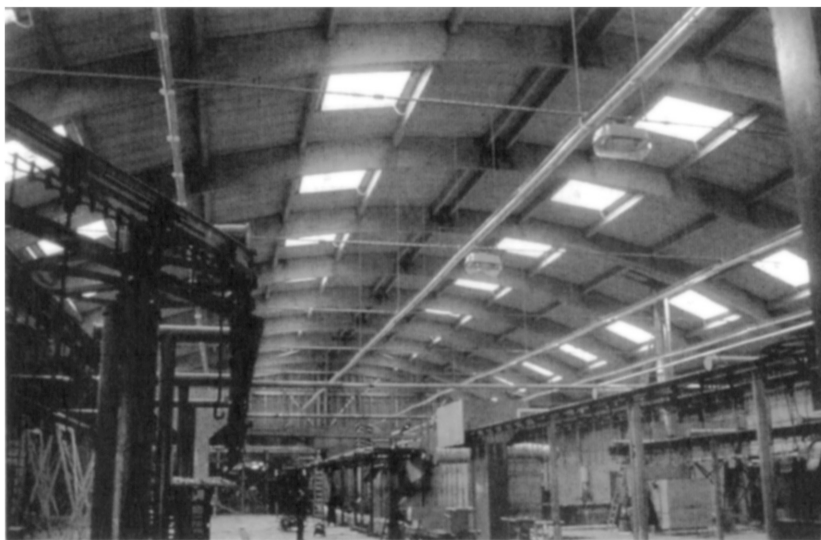
Figure 5 Timber roof structure of an enamel smelting house.
