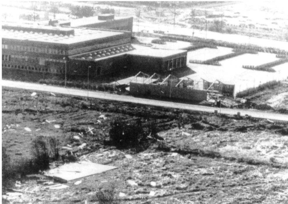
Figure 8 View of the damaged building. A blown-off roof section can be seen to the left.
