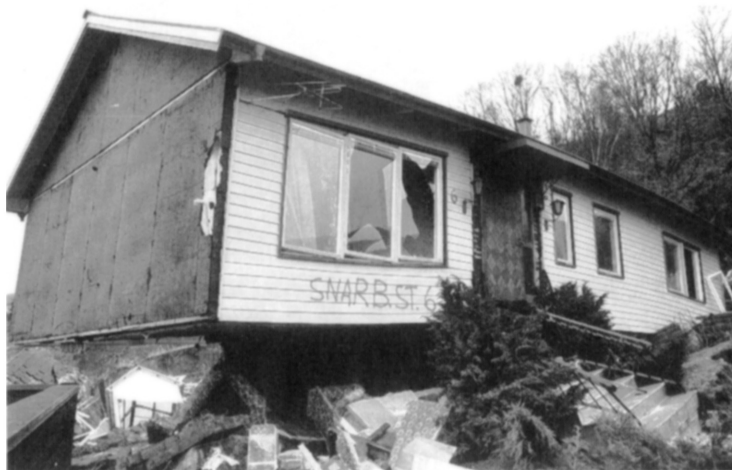
Figure 25/26 The house rests only on the centre walls and cantilevers in all four directions. Notice the shear deformation in the window openings.
