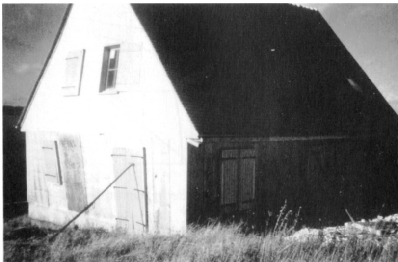
Figure 10 Instability of timber frame walls.
