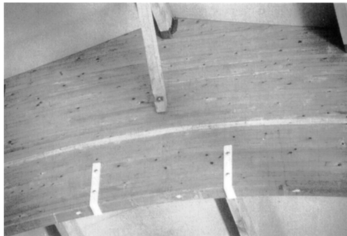
Figure 13 Cracking of tapered curved beam.
