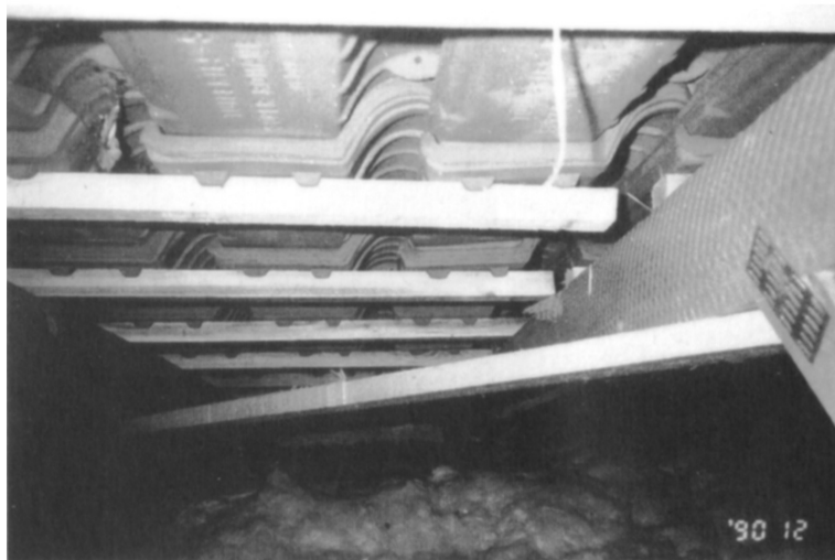
Figure 7 Slipping and dragging of batten nailing.
