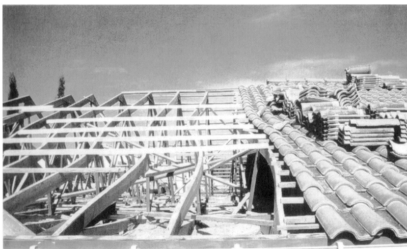
Figure 6 Buckling of trussed rafters.
