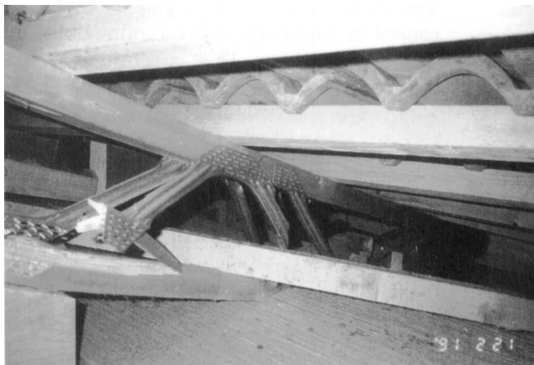
Figure 8 Failure of timber girder.
