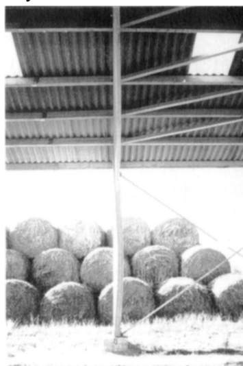
Figure 9 Warping of LVL frame.
