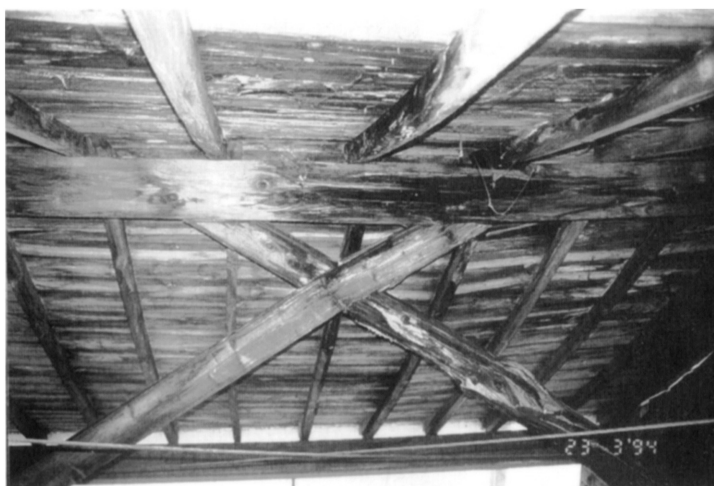
Figure 5 Serious damage by fungus.
