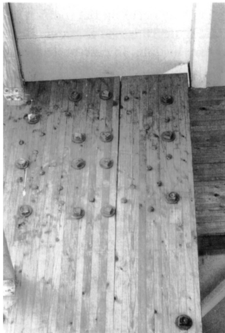
Figure 19 Cracked frame corner.
