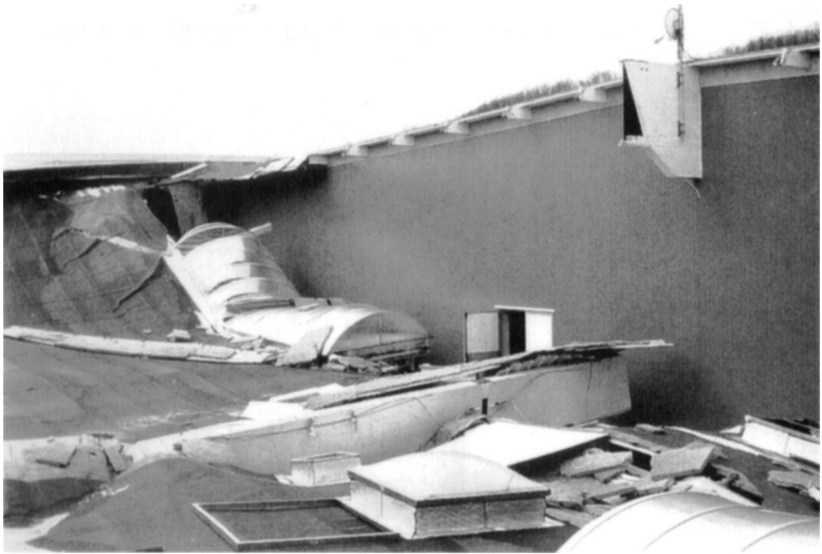
Figure 20 Failure of cantilever joint.
