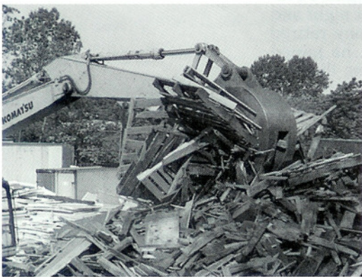
Pallets are crushed with an excavator grapple and sent to a colored mulch producer.
