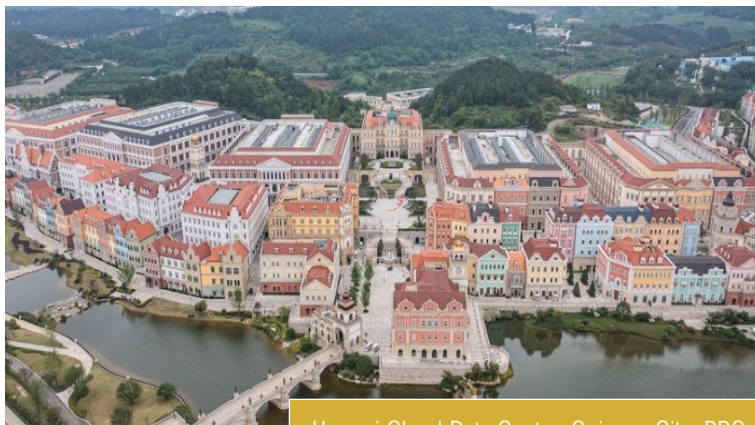
Huawei Cloud Data Centre, Guiyang City, PRC
