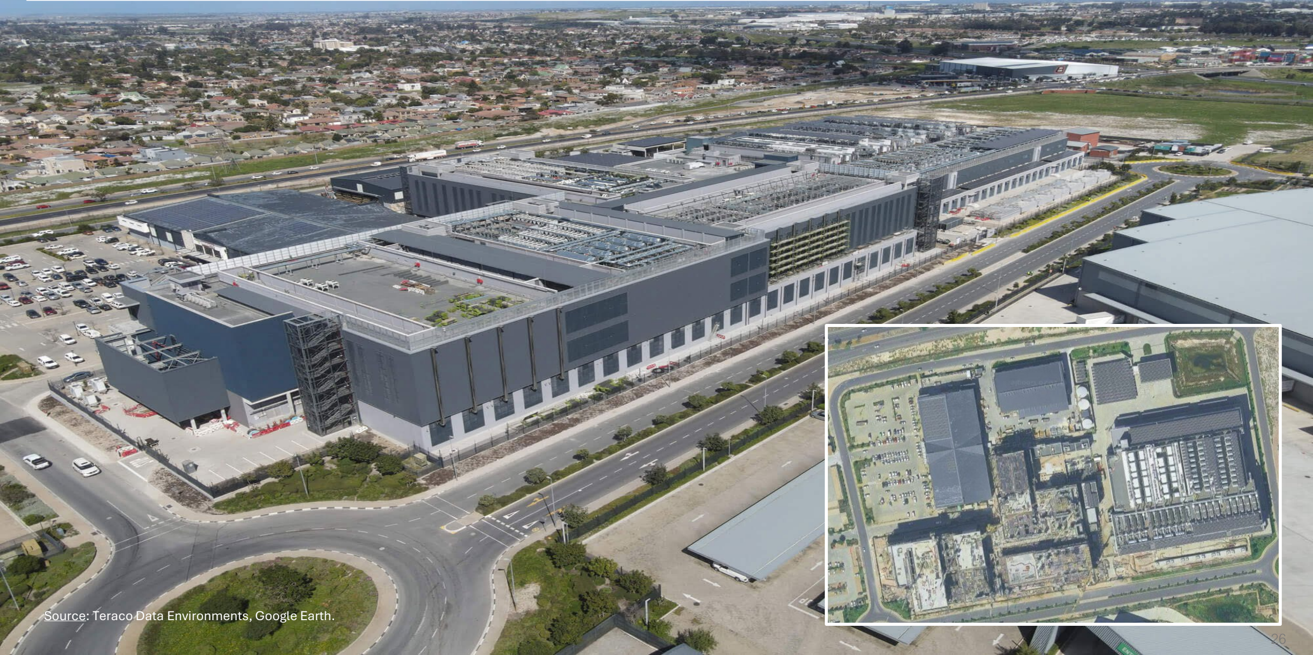
Teraco Data Environments, CT2, Brackengate 2, Brackenfell, Cape Town, 50MW.
