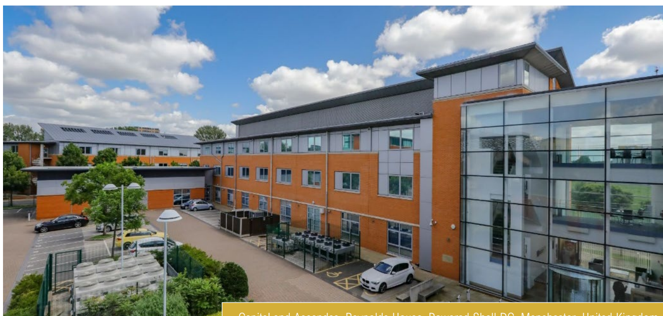
CapitaLand Ascendas, Reynolds House, Powered Shell DC, Manchester, United Kingdom
