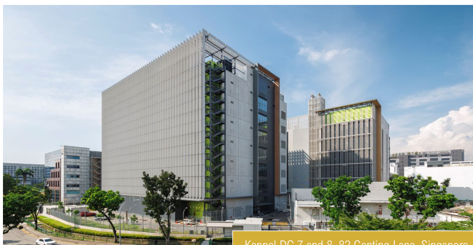
Keppel DC 7 and 8, 82 Genting Lane, Singapore
