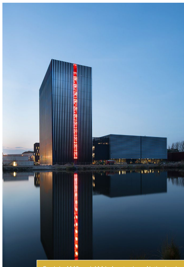
Equinix AM3 and AM4, Amsterdam, Netherlands
