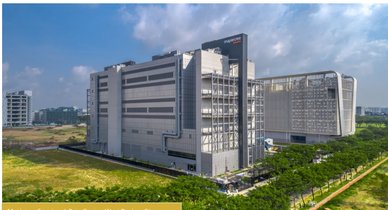
Mapletree Sunview 1 Data Centre, West Region, Singapore
