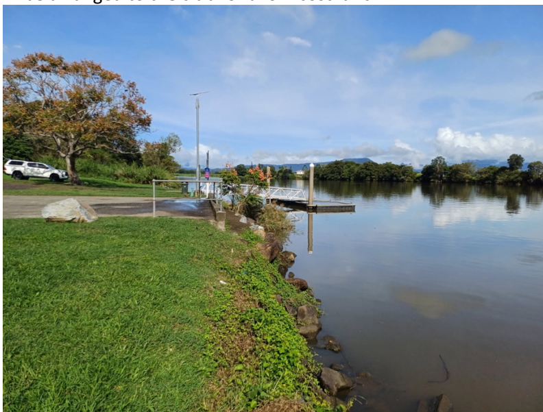
Condong Boat ramp
