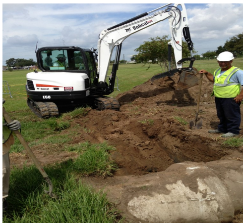
Drainage line point repairs NASA Michoud Assembly Facility
