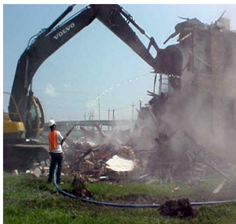
New Orleans Ninth Ward Demolition Ninth Ward Redevelopment Association
