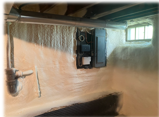
Foam was sprayed on the basement walls to insulate and prevent deterioration of the stone.
