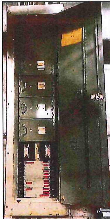
Examples of existing electrical panels from school (left) and boiler room (above). These outdated systems require replacement and new wiring to upgrade.
