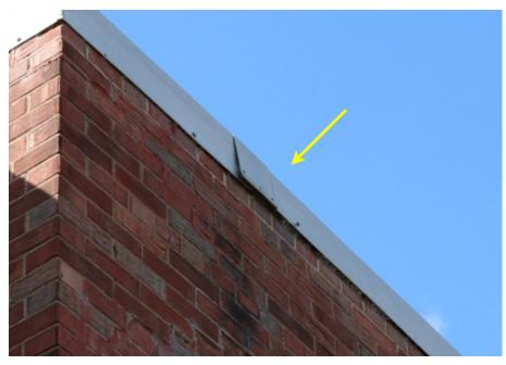
Several conditions observed in the roof perimeter cap system are likely having an impact on the masonry wall below. One of the most obvious conditions is that several of the cover plates between cap sections are coming loose.
