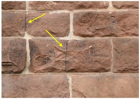
Narrow stone cracks like those pictured here can often be repaired using a combination of epoxy injection and surface patching.
