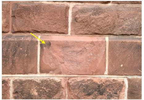
The condition where outer layers of a stone flake off is known as "spalling". When the depth of the spalling is not too severe, it is sometimes possible to remove the stone and recarve the surface profile before reinstalling it. This is an especially useful option when working with historic stone that is no longer available from any quarries.
