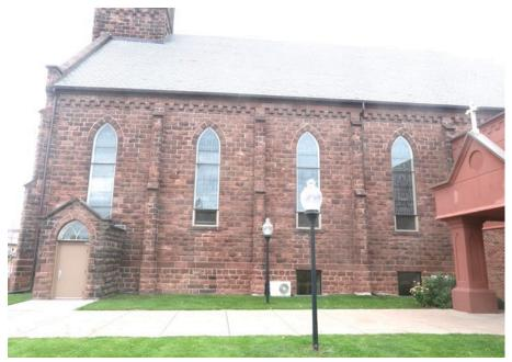
The east side of the church is also included in the attached budget estimate. We are recommending that 100% of the mortar joints be cut and tuckpointed as part of the work, but it is not possible to accurately predict the quantity of stone repair and replacement that will be needed until the work is under way. The estimate includes unit prices for this type of work item where the actual quantity can vary.
