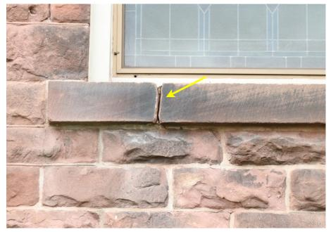
This close-up shows the opening in the sill stone. When the original mortar cracking was noticed, if the repair had been done properly it is unlikely that the crack would have spread to the point where the sill was cracked.
