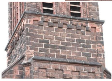
A noticeable feature of the church is that the stone exterior is badly soiled. Costs for chemical cleaning of the building are included in the attached budget estimate.
