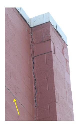
Vertical cracking in the block wall sections of the building appears to be related to the lack of flexible control joints. The severe deterioration visible at the upper corner is typical of the damage caused by repeated cycles of freezing and thawing when the masonry is saturated. The full repair of this condition will likely require some work at the connection between the roofing and the masonry.
