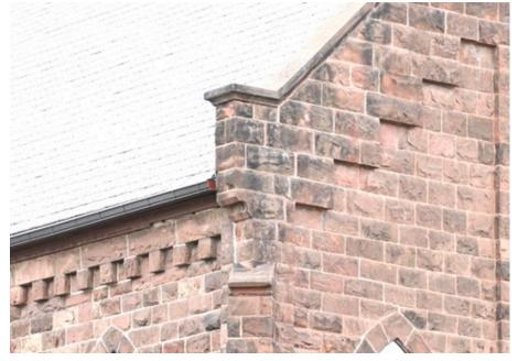
In 2015, loose stones were reset and anchored on both ends of the main gable wall. The stones appear to be stable as there are no signs of shifting or cracking of the masonry on either corner.
