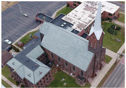
Masonry repair and maintenance is needed on all of the Our Lady of the Lake campus buildings. Cutting and tuckpointing of deteriorated mortar joints, patching and replacement of damaged stone and bricks, removal and replacement of caulking sealant, and other related work is outlined in this report and the attached budget estimate.
