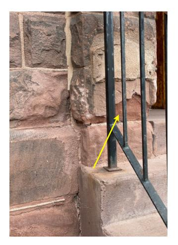
Examples of different types and degrees of stone damage are shown in these photos. Conditions run from weathering away of the stone surfaces to deep cracking and loss of portions of the stones. Recommended repairs depend on the individual stone conditions. In some cases, cutting back and replacing the surrounding mortar is a reasonable response. In other cases, entire stones may need to be replaced because the existing ones are too badly damaged to be repaired.
