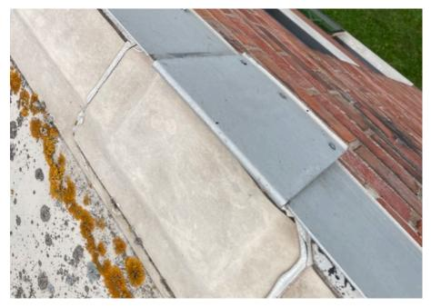
Sealant joints in the roofing system are weathered to the point where they may no longer be providing protection against water infiltration to the building components below. The condition of the roof should be verified as part of any masonry repairs to the walls below.
