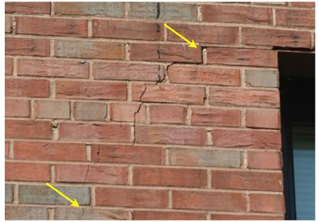
During the course of repairing this crack, a number of brick will be removed from the wall. This will provide on opportunity to see the construction detail and some of the interior wall conditions.
