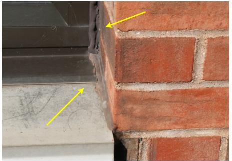
The window perimeter caulking sealant shown here is cracking and no longer providing protection against water infiltration. Also, the staining on the grey aluminum sill suggests that the sill is pitched back towards the building allowing water to pool at the joint with the window frame.
