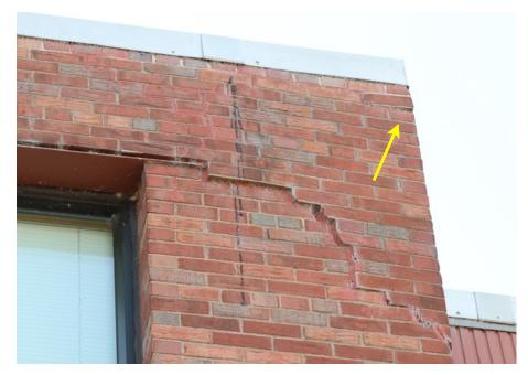
In addition to the stair step cracking pattern seen at several other windows on the building, there are displaced bricks at the top of the highlighted corner.
