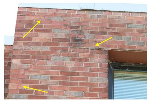
The cracking highlighted here is likely caused by the pressure from the build up of flaking pack rust on the window lintel. Close observation of this lintel showed that it has bowed down in the center. As a result, the ends of the lintel are lifting the brick to the left of the opening. The pressure is severe enough to break the bond of the mortar joints creating a typical "stair step" cracking pattern.
