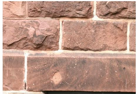
There are many examples of poor quality work on the building. Not only does the mixture of mortar colors and joint profiles look bad, it is obvious that this type of work is bad because the "repairs" have failed so quickly.
