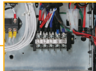
Outdoor unit power supply terminal block
