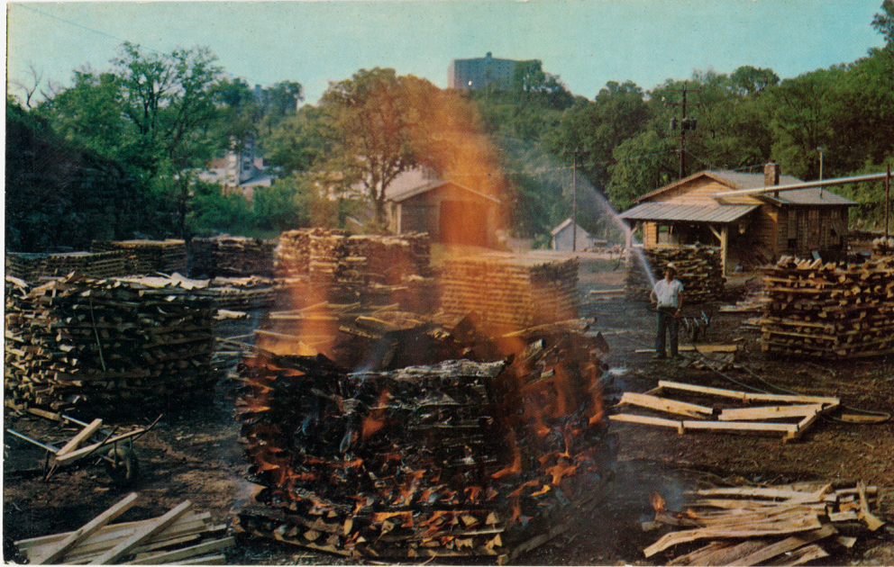
Jack Daniels Rick Method. Making charcoal for the Jack Daniels Distillery using open ricks (photo: Wikipedia).
