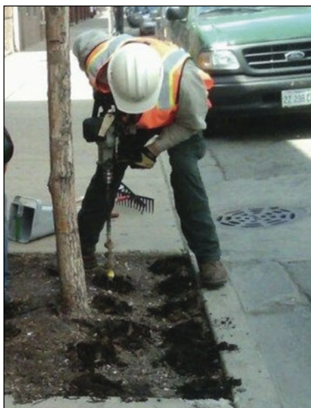
Auguring holes for biochar applications to street trees in Bucktown, Chicago, Illinois. Courtesy of Bryant Scharenbroch/Morton Arboretum Soil Science ( www.masslaboratory.org ).
