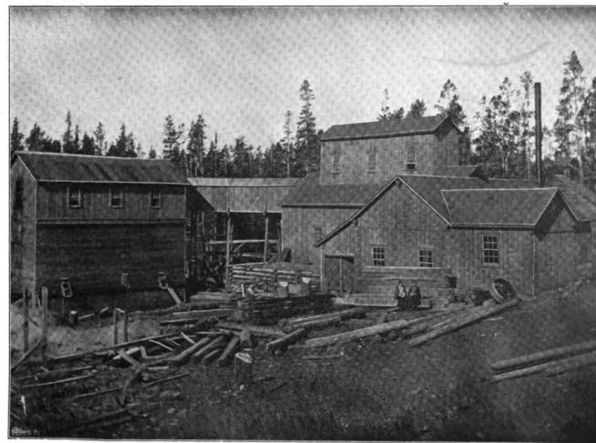
NEW RAMBLER MINE SHAFT HOUSE.
