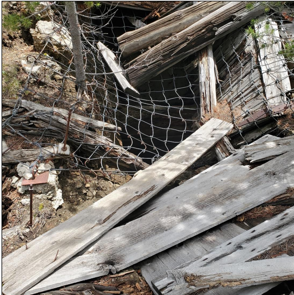
Joker No. 4 Lode, timbered mining shaft (~135 ft deep)
