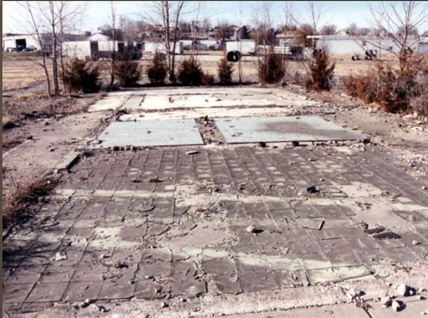
50 HIWA Drive In – Projection Booth Foundation (in 2002)
