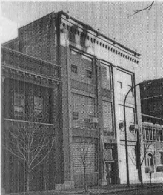
2309-2311 Locust Willys-Overland Building
