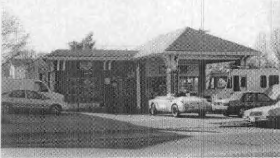
Gas Station 6300 Block of Arsenal
