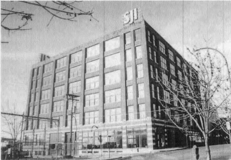
2300 Locust, Willys-Overland Building
