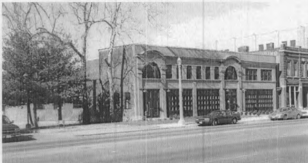
Service Garage 2337-2345 S. Grand
