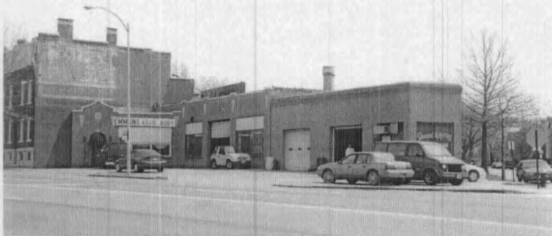
Service Garage 2230 Gravois
