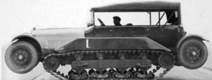
This 1926 Wolseley-Vickers car was equipped with both tracks and regular wheels so the vehicle could be driven around like a traditional car or it could lower its tracks to tackle rougher terrain like a tank.
