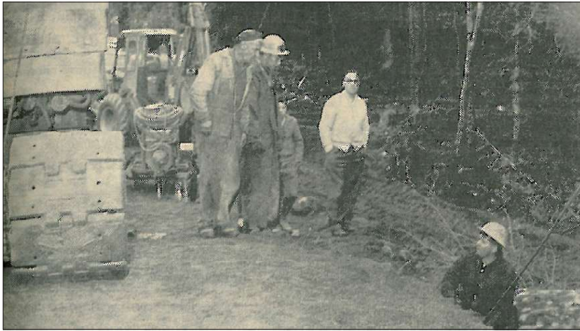
Bridge builders anchor the stringer cables across the Coquihalla River on the golf club bridge in May 1964.
