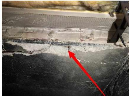
**FIRE DRFT 17: Breast Plate: Exposed Rebar**
