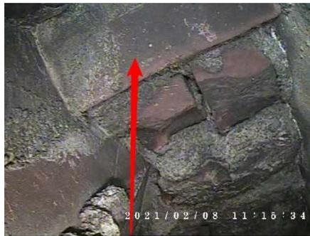
**FIRE DRFT 21: Smoke Chamber: Gaps At The Transition To The Flue Liner**
