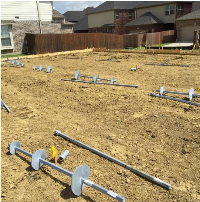
Triple-Helix Helical Piers are laid out on the job site in preparation for installation
