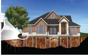
Designed to perform as a suspended slab, Tella Firma provides the strength of a pier-and-beam foundation system, yet is much more affordable and takes less time to install than most traditional suspended foundations.
