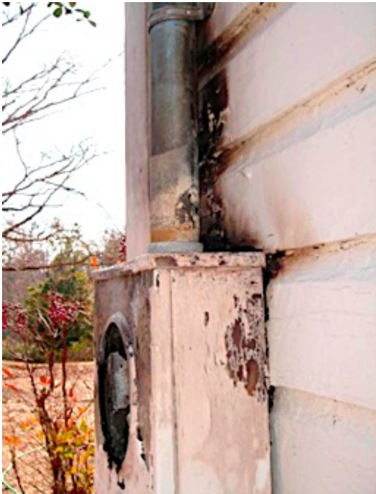
(a) Localized, but limited burn damage to wall
