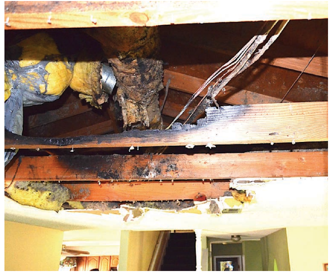
Figure 78 Fire originating mid-run on a branch circuit, about 3 – 4.5 m away from a smart meter which was installed some 4 – 6 months earlier. Examination of the fire origin area did not reveal any fasteners that could have damaged the cable, nor any other potential sources of mechanical damage. (Photo: Jim Brown)
