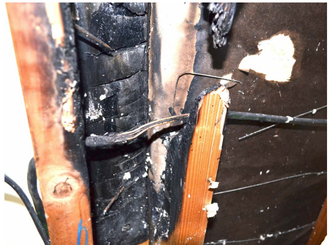
Figure 79 Fire originating in a wall cavity causing heavy damage to two studs. The smart meter was located about 4.6 m away. No arc marks were found on the NM cable. No staples, nails, or other mechanical causes of damage were found. The photo also shows some bare wires which were part of the wall stucco construction method. (Photo: Jim Brown)
