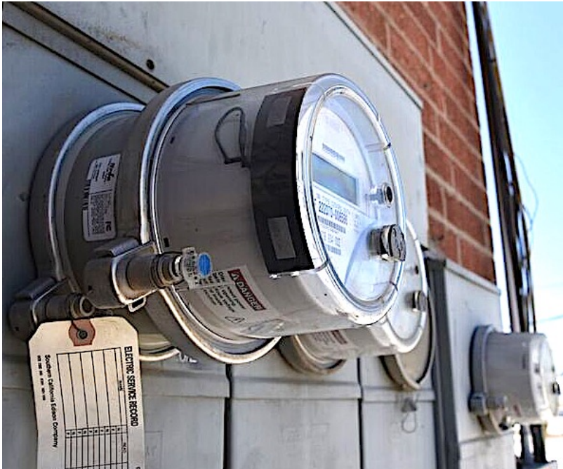
Figure 74 Smart meter installation, showing two ordinary smart meters (center, right), and a collector meter (left). Note that the collector meter differs in having an extra-deep base.
