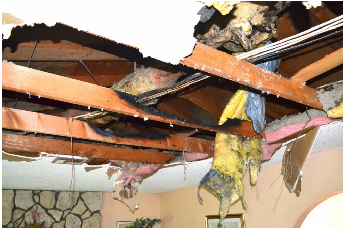
Figure 80 Fire originating mid-run on a branch circuit, about 3.9 m away from a smart meter which was located on the exterior face of the wall along the left side of photo. Note two joists with extremely heavy saddle burns, while no damage was seen to adjacent joists. No staples, nails, or other mechanical causes of damage were found. (Photo: Jim Brown)
