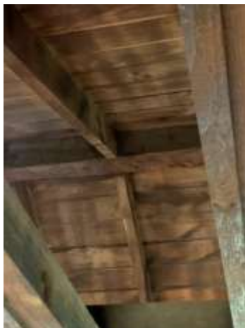
Figure 13. In the reconstructed log schoolhouse, the center roof rafter of the Norman truss , is an original 1837 log.
