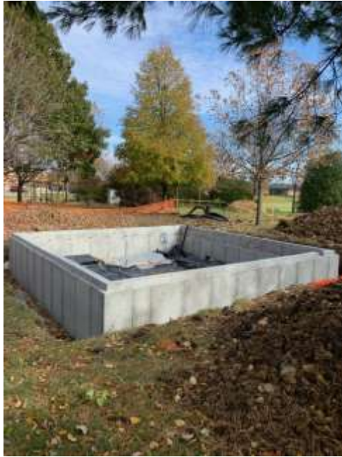
The log schoolhouse foundation is complete—November 16.
