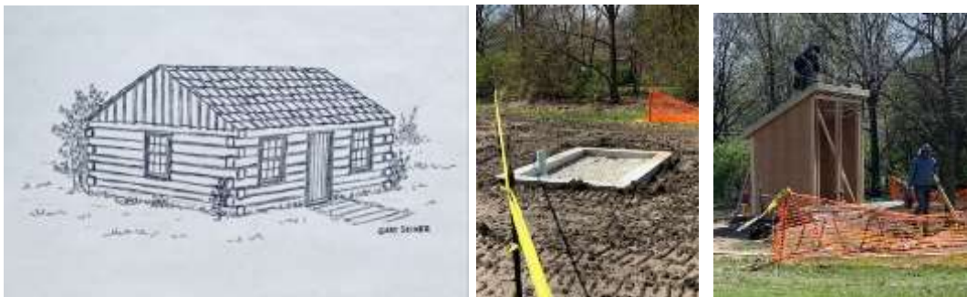
Pictured: (from left to right) Gary Seiner’s recent drawing of the log schoolhouse, pad of “outhouse” (utility building) with buried HVAC lines, and April 26 framing of outhouse.
