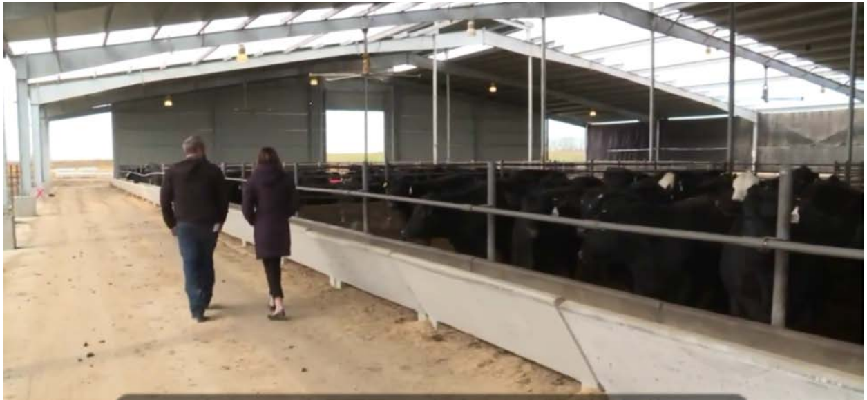
Photograph 2. Stem Walls at Valley Oaks CAFO.
