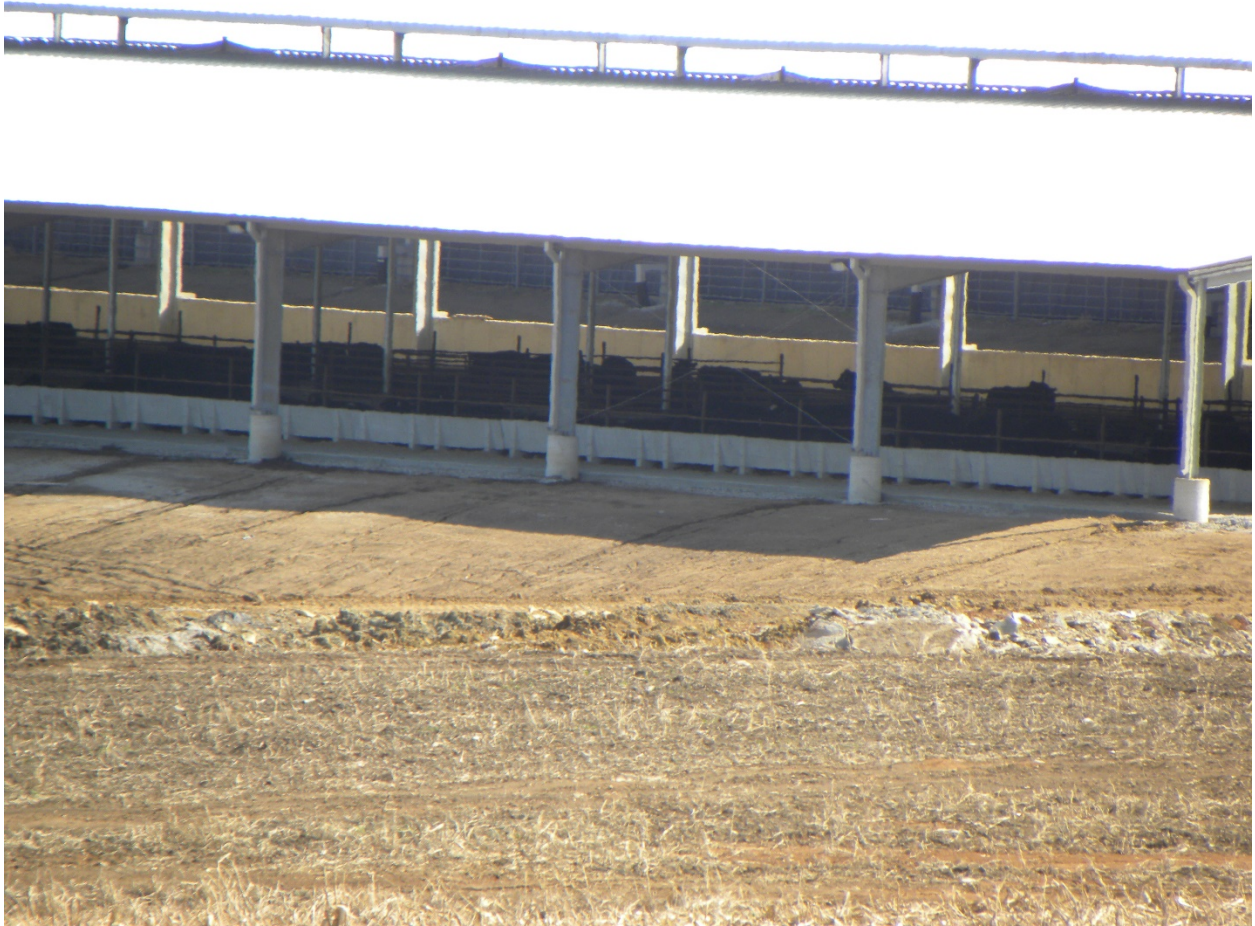
Photograph 1. Stem Walls at Valley Oaks CAFO.
