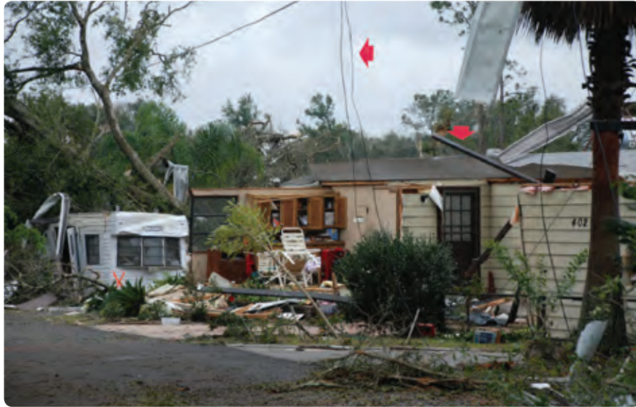
Figure 23-2. Check the scene for dangers that could threaten your safety or the safety of others, such as downed wires and unstable structures.
