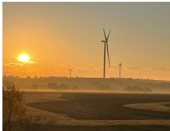
Windmills at ENGIE's Priddy Wind Project in Texas
