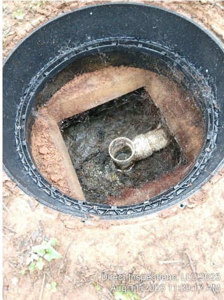
Tank access and input baffle
