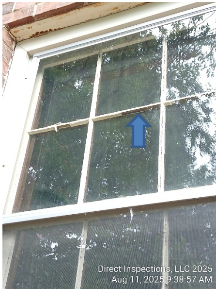
Glazing deterioration
