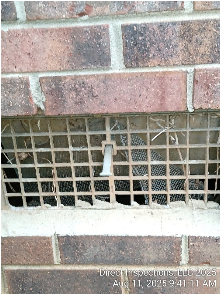
Damaged screen
