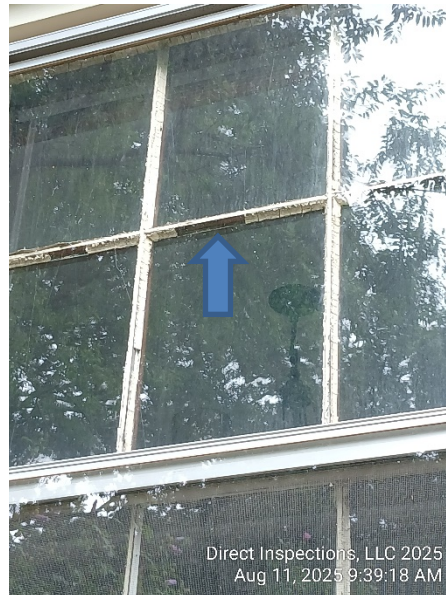
Glazing deterioration
