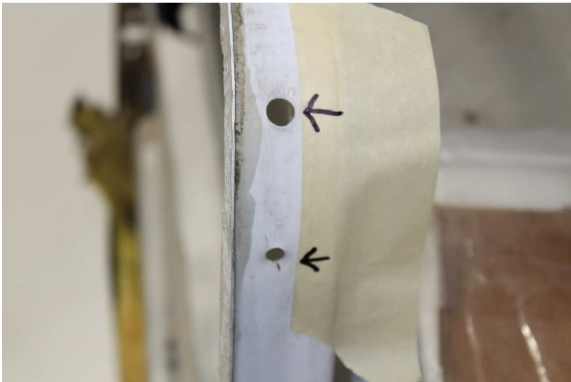
Accommodating for Window Assembly
