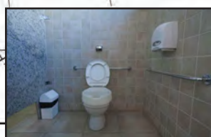
Upgrading bathrooms to ADA compliance.
