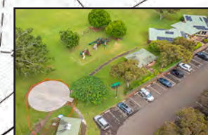
The FitLot under construction
