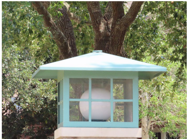
Metal roof and light fixture overview
