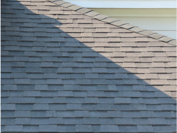
Pool house asphalt shingle roof overview
