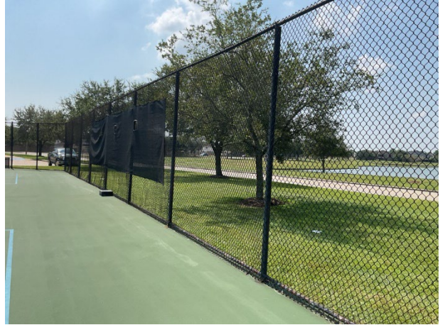
Chain link fence overview
