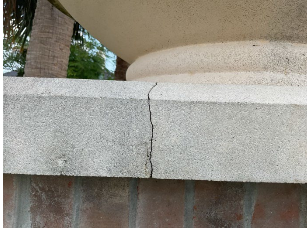
Concrete cracks
