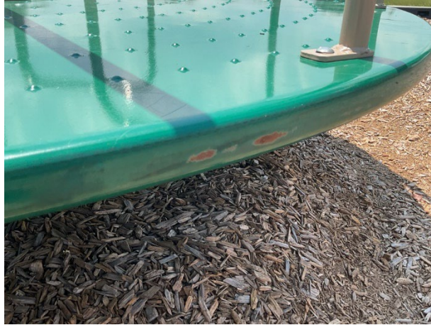
Frame rust at Woodcock Street
