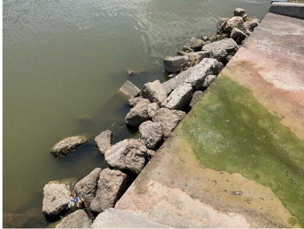
Stone rip rap overview
