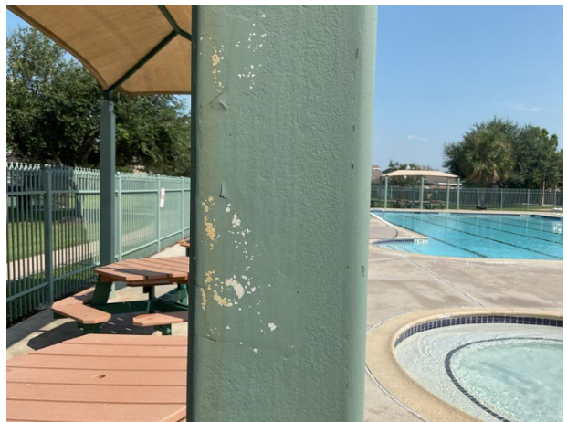
Finish deterioration
