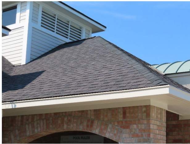
Pool house asphalt shingle roof overview
