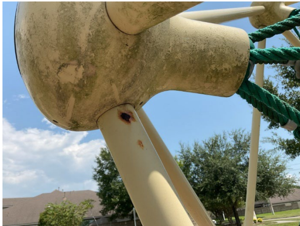
Frame rust and organic growth at Brook Arbor Lane
