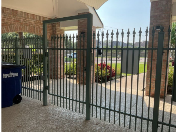
Metal pool fence gate overview
