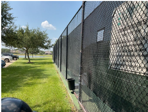
Chain link fence overview
