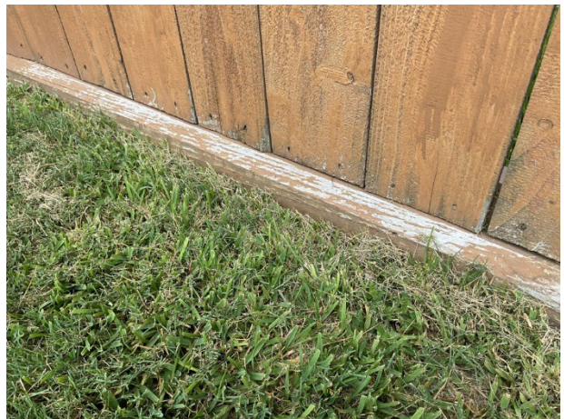
Finish deterioration
