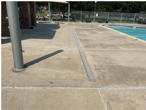
Concrete pool deck overview
