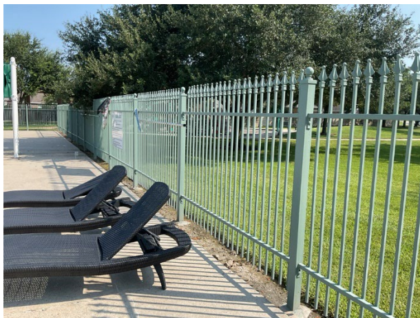
Metal pool fence overview
