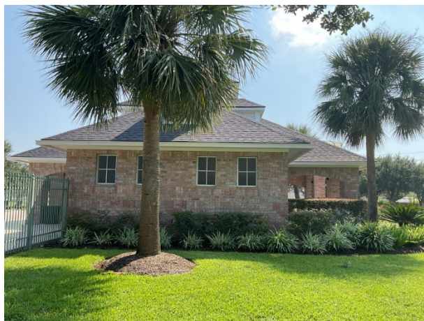
Side elevation overview
