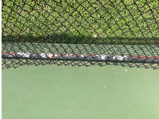
Finish deterioration
