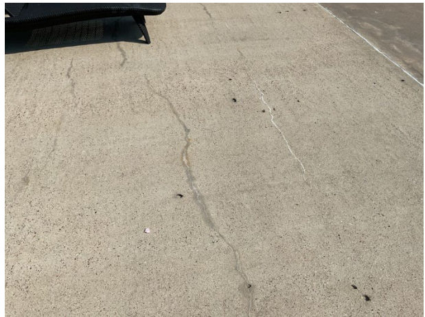
Concrete pool deck overview
