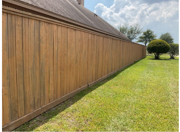
Wood fence overview
