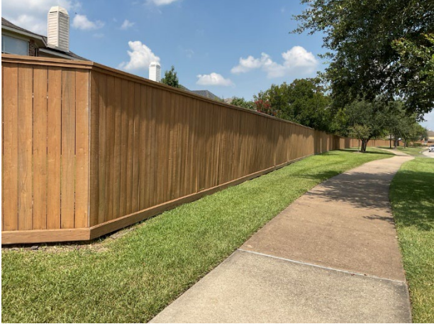
Wood fence overview
