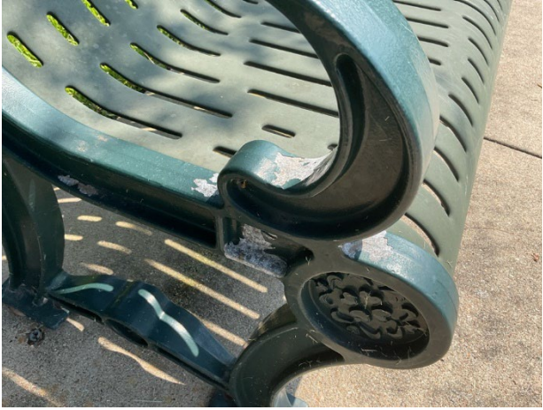
Finish deterioration
