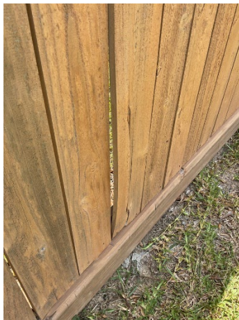
Warped wood
