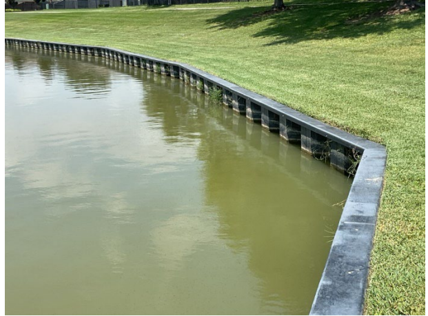
Vinyl bulkhead overview
