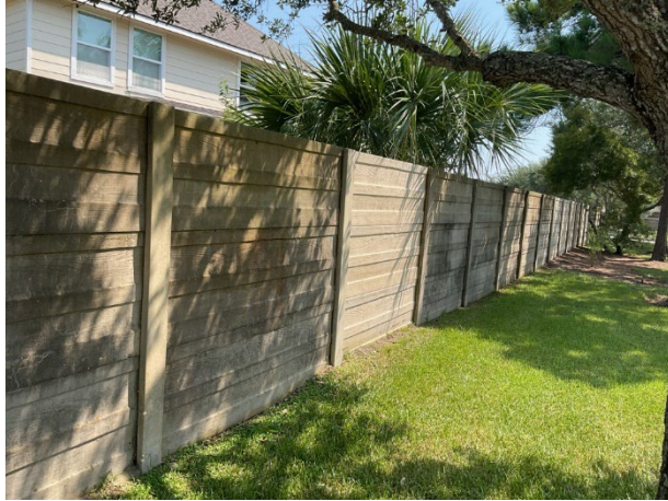
Concrete perimeter wall overview
