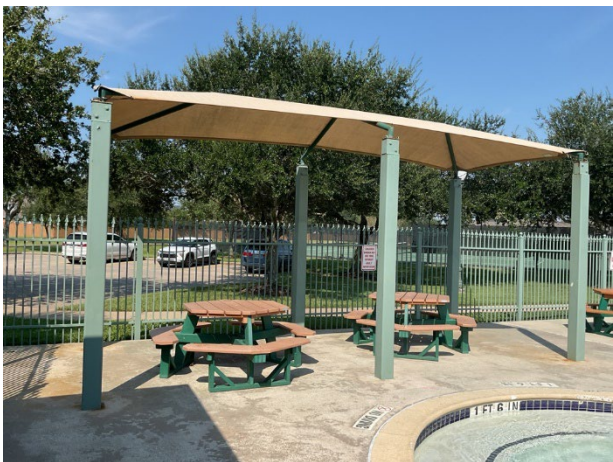
Shade structure overview
