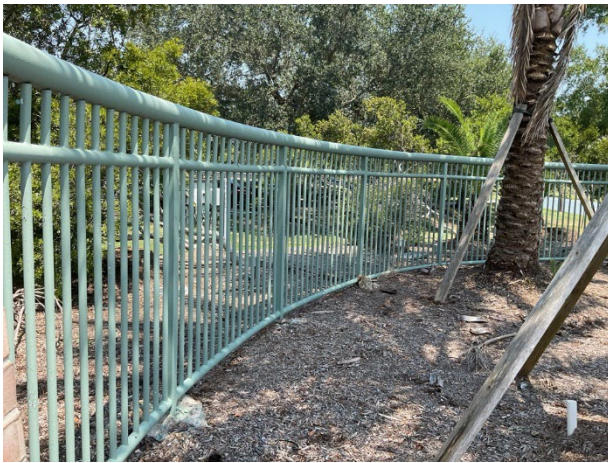
Metal railing overview
