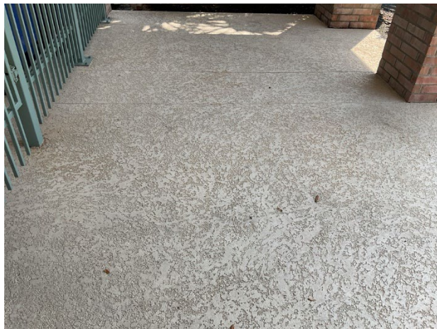
Concrete floor overview
