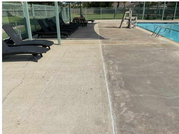
Concrete pool deck overview
