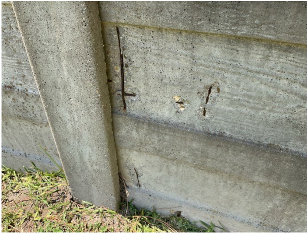
Exposed reinforcements
