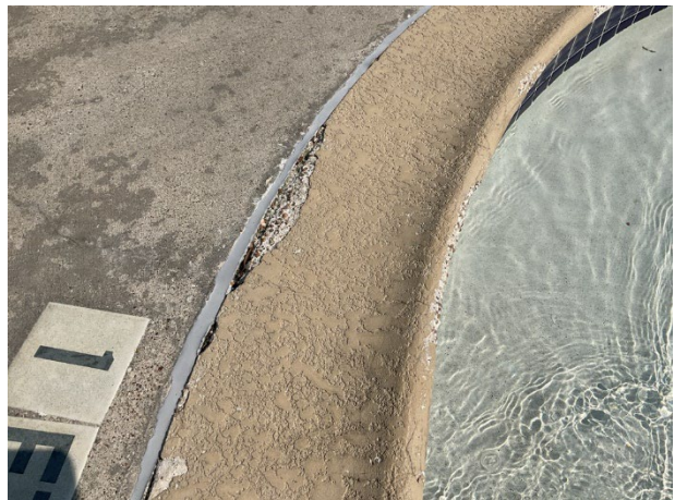
Coping deterioration
