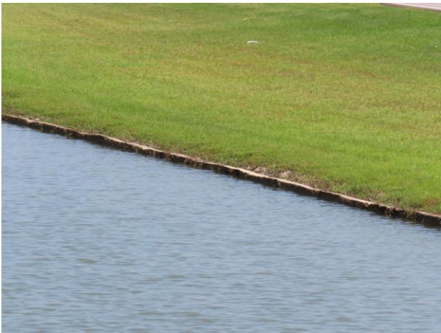
Entrance bulkhead overview
