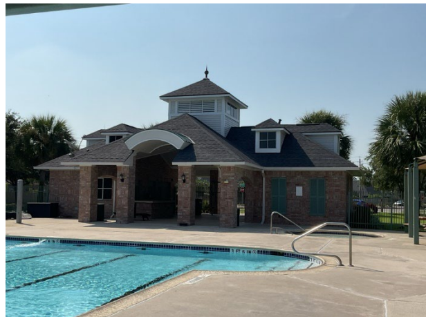
Rear elevation overview
