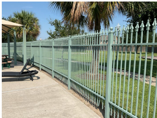
Metal pool fence overview
