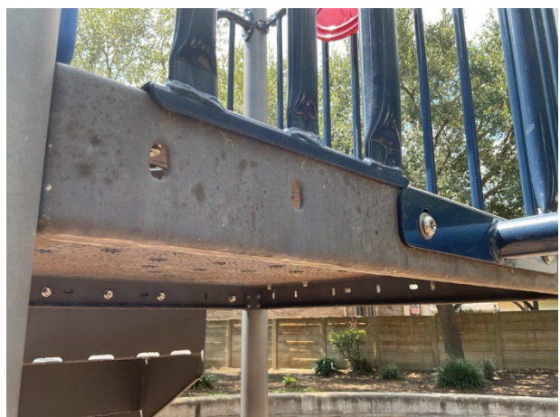
Equipment finish deterioration at Island Crossing Lane
