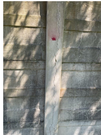
Concrete cracks
