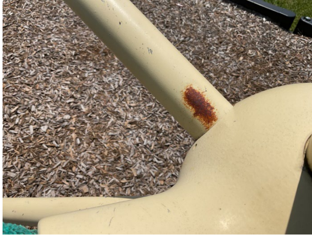
Frame rust at Brook Arbor Lane
