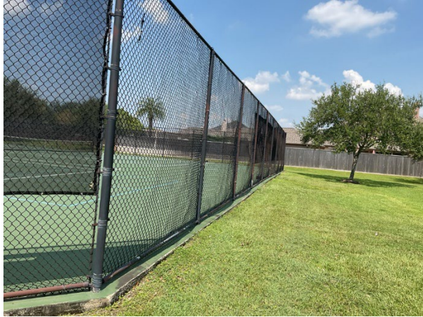
Chain link fence overview
