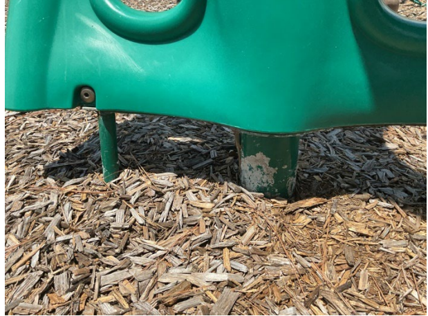
Equipment finish deterioration at Brook Arbor Lane
