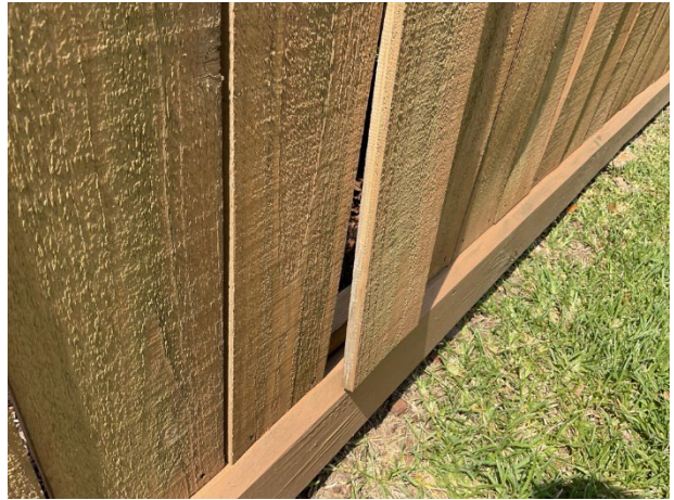
Warped wood
