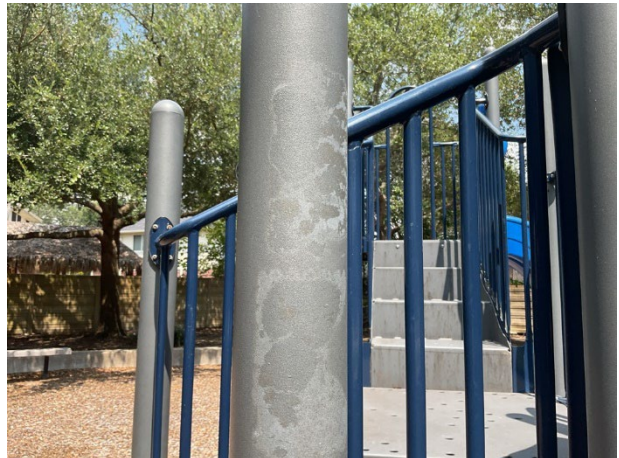
Equipment finish deterioration at Island Crossing Lane
