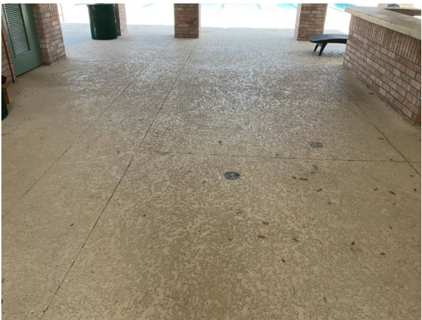
Concrete floor overview
