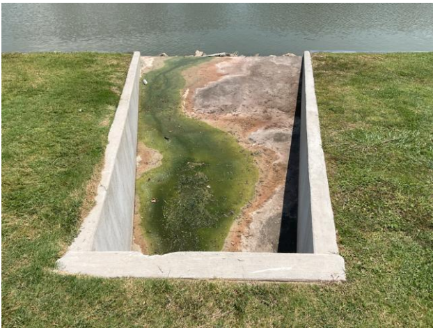
Concrete inlet/outlet structure overview
