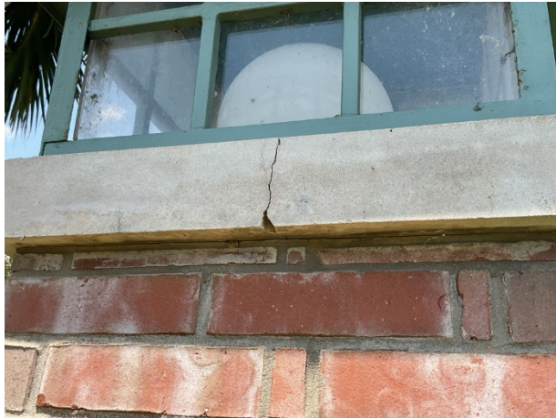
Concrete crack
