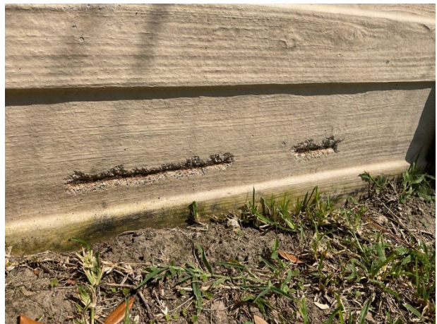
Exposed reinforcements
