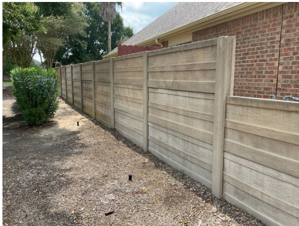
Concrete perimeter wall overview
