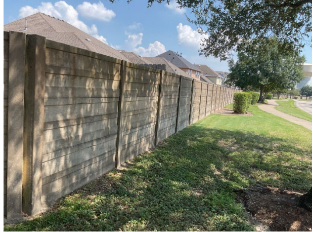
Concrete perimeter wall overview
