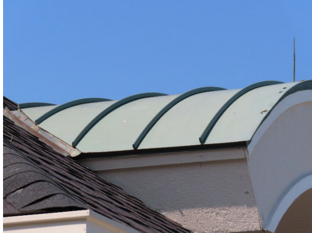
Metal roof overview
