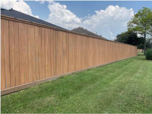
Wood fence overview
