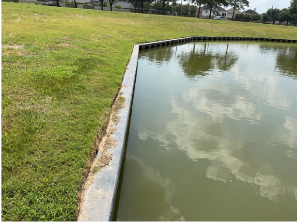
Vinyl bulkhead overview
