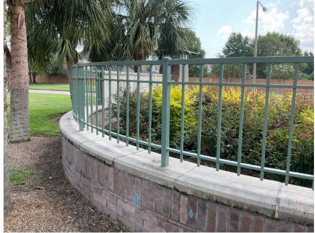
Metal railing overview
