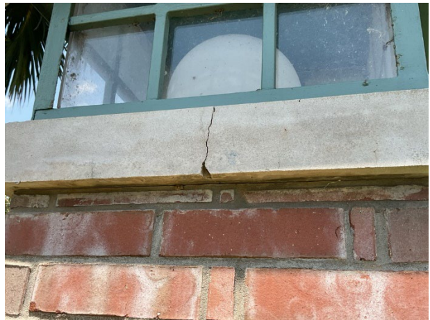
Concrete crack
