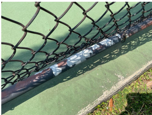
Finish deterioration
