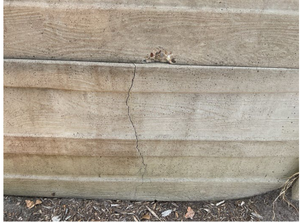
Concrete cracks
