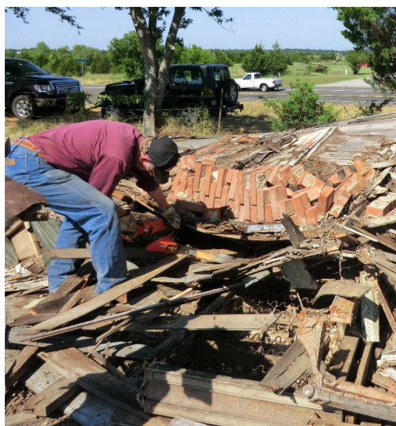
Alan using his chainsaw to help clear the debris left by the collapse of the superstructure at the Redwine Site (41COL228).
