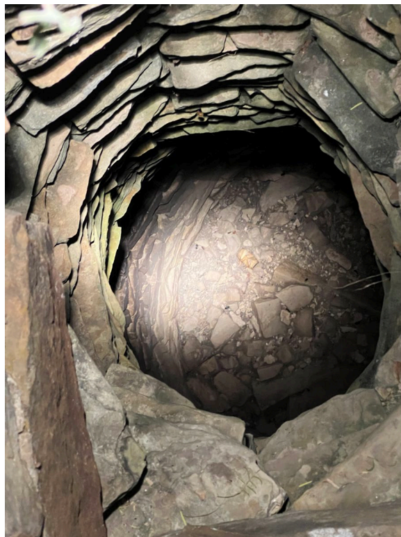
Figure 6. Photo taken at night using artificial light looking into the cistern.
