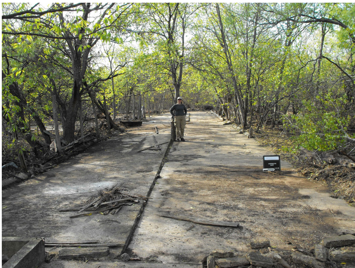
Figure 10. Milking parlor, view facing west from rooms A and B. Pour line of slabs is visible in center of foundation, while standing cedar post are seen in the background.
