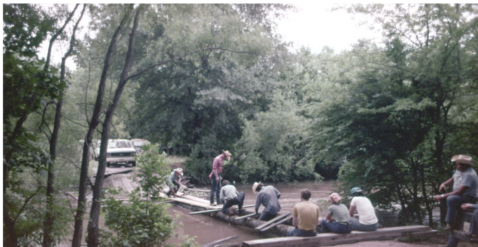
A series of photos of Alan(in the red shirt) instructing others on how to build a bridge during the Lake Fork Reservoir Project. Photos credit: ARC@SMU.
