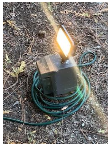
West SSL - New LED floodlight
