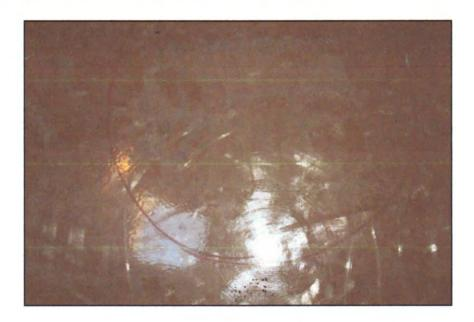
PHOTO (5) You can see the scratches in the coating, the floor was supposed to have been clean of all dirt but was not. The tank erector was not on site and had left the state.
