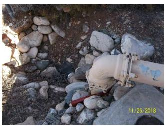
Storage tank overflow is not 12 to 18 inches above ground.
