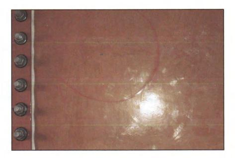
PHOTO (2) One of the reasons for so many holidays is the coating is thin 5.7 mils and scratches easily. A normal coating on a potable water tank interior is 10.5 to 12.5 mils DFT
