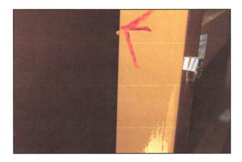
PHOTO (4) This is a ladder rung or angle used for the ladder with holidays on all the ends of the angle used for the ladder.
