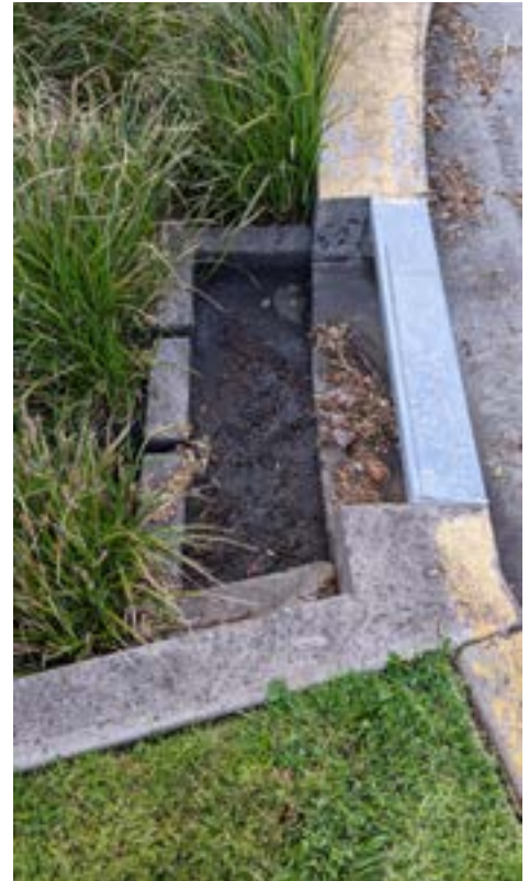
Pre-treatment Sediment Drop with sediment build-up.
