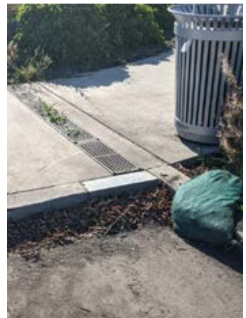
Facility inlet clogged with leaf debris.
