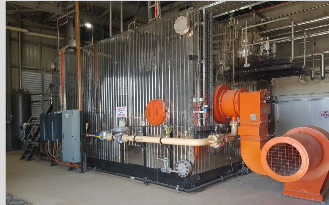
10 Mw 42 bar steam boiler commissioning Australia
