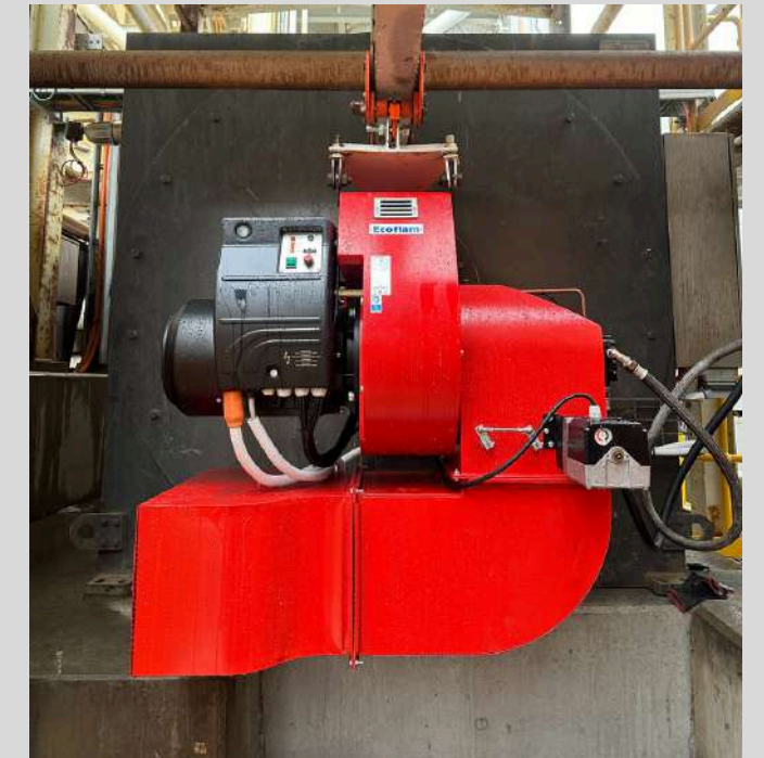
5000 Kw burner upgrade Laos
