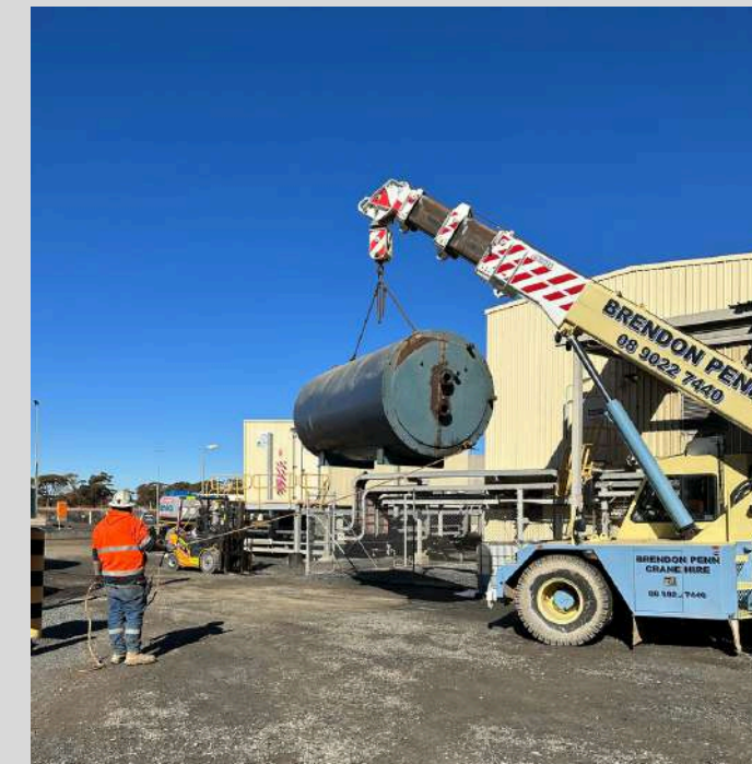
Elution heater upgrade West Australia
