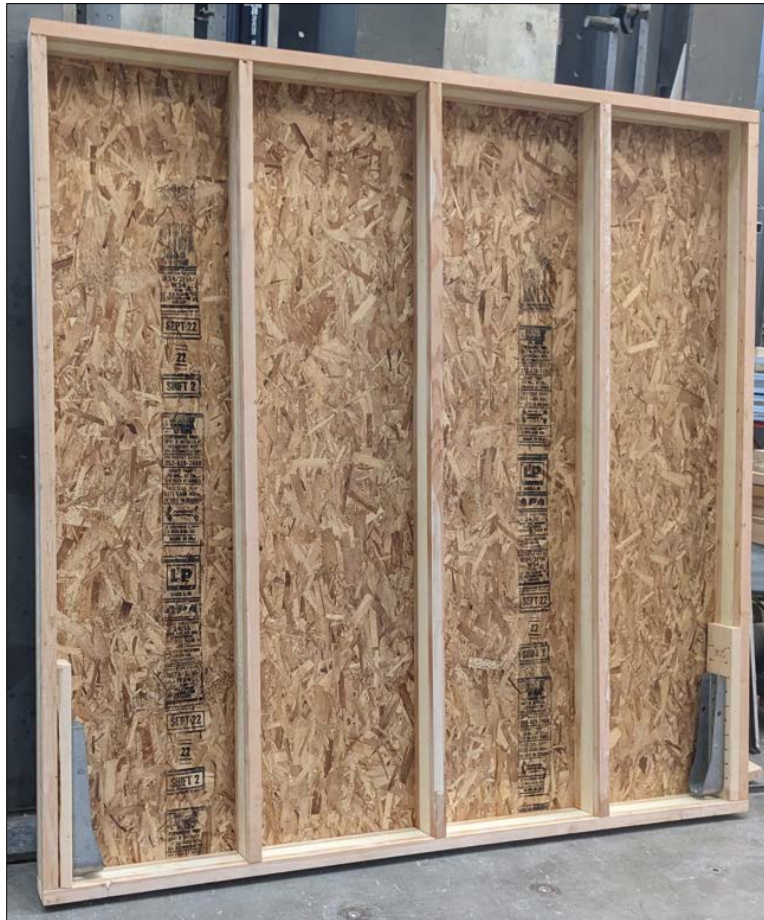
Figure 2. Insul-Stud Structural Insulated Stud Wall Assembly
