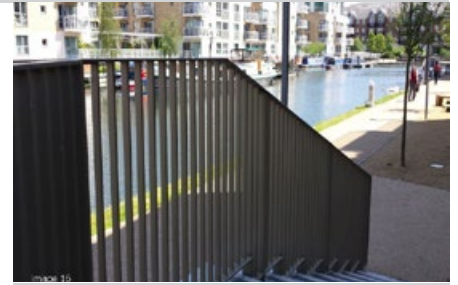
MODERN 1C Vertical infill all 1" square tube
