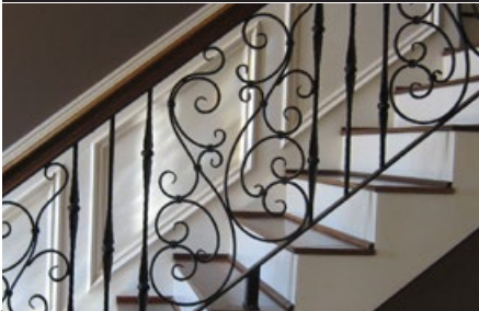
TRADITIONAL 4A 9/16" Gothic square hammered bar scrolling HF16.1.8, HF16.5.2, 3/4" flat bar scrolls
