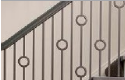
TRANSITIONAL 2A 1/2" plain square bar with Aalto circles HF16.2.1, HF16.1.30, HF16.1.31
