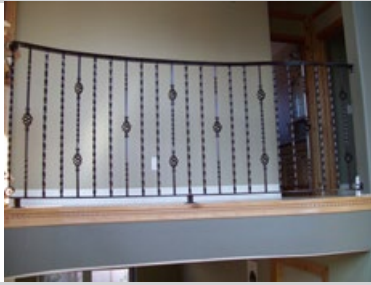
TRADITIONAL 1B 1/2" plain square bar w/ twists & baskets. HF16.1.3, HF16.1.4, HF16.1.21
