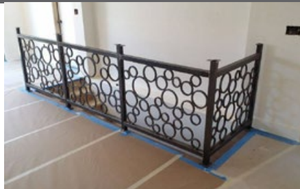
CONTEMPORARY 3B random geometric shapes - 1/2" square solid bar
