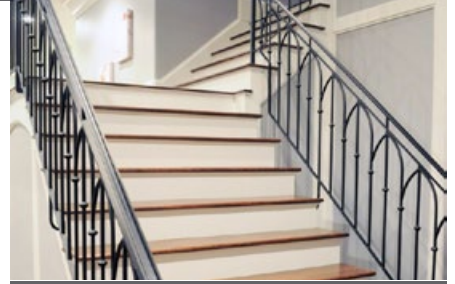
TRADITIONAL 3C 1/2" plain square bar/knuckle w/ subrail custom scrolls
