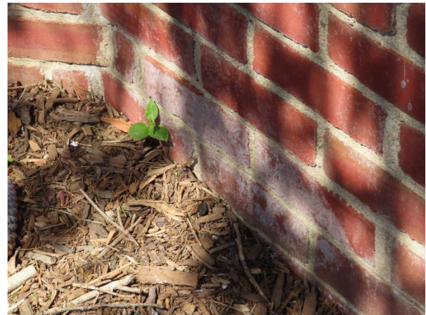
Efflorescence
