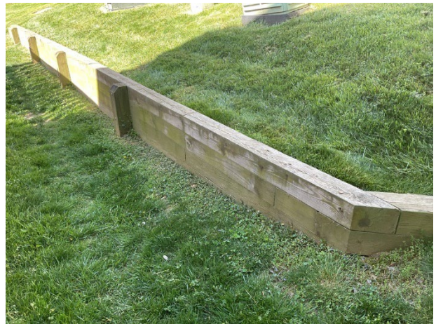
Timber retaining wall next to 9433 William Kirk Lane
