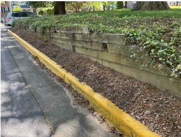
Timber retaining wall on Peter Roy Court
