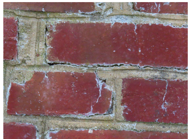
Mortar cracks
