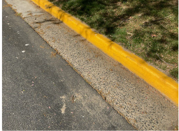
Concrete spalls
