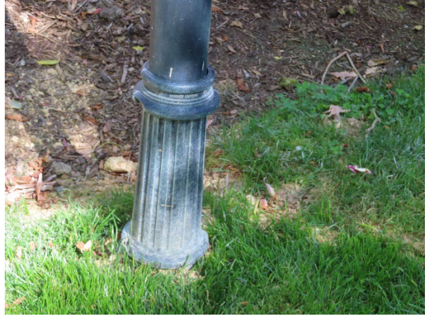
Finish deterioration
