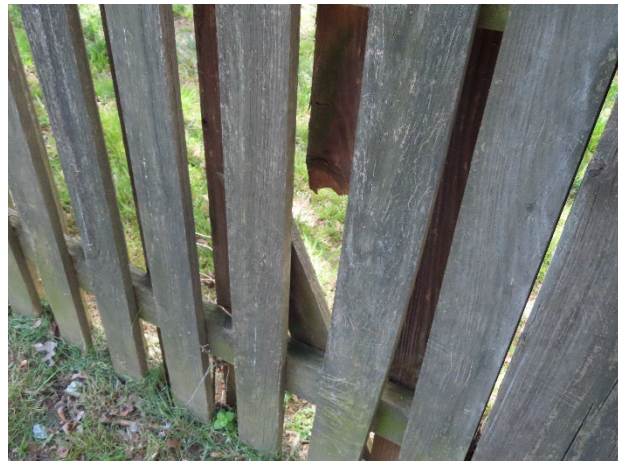
Damage to wood fence
