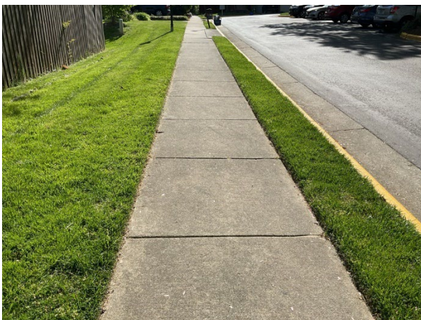
Concrete sidewalk overview
