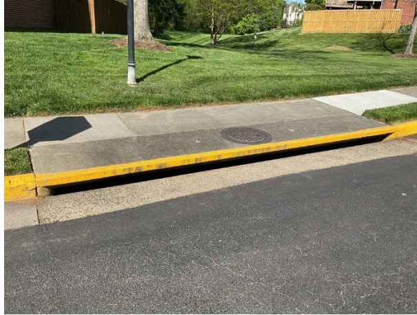
Catch basin overview
