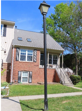
Leaning light pole
