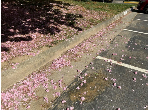
Concrete curb and gutter overview
