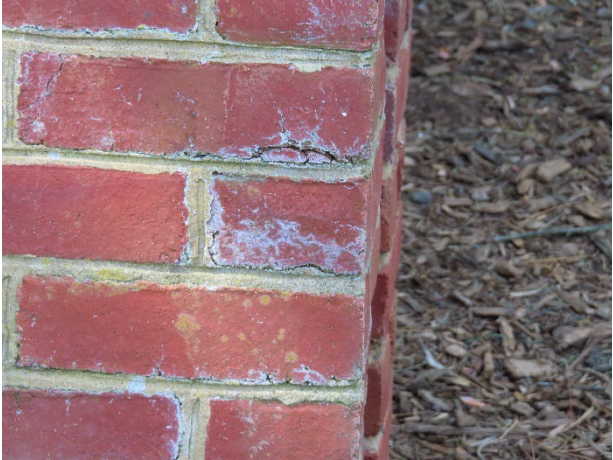
Masonry cracks
