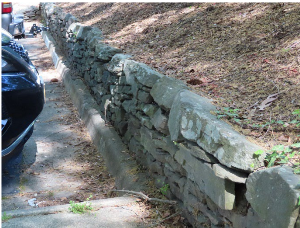
Stone retaining wall overview
