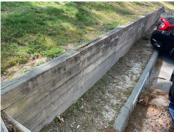
Timber retaining wall on Peter Roy Court
