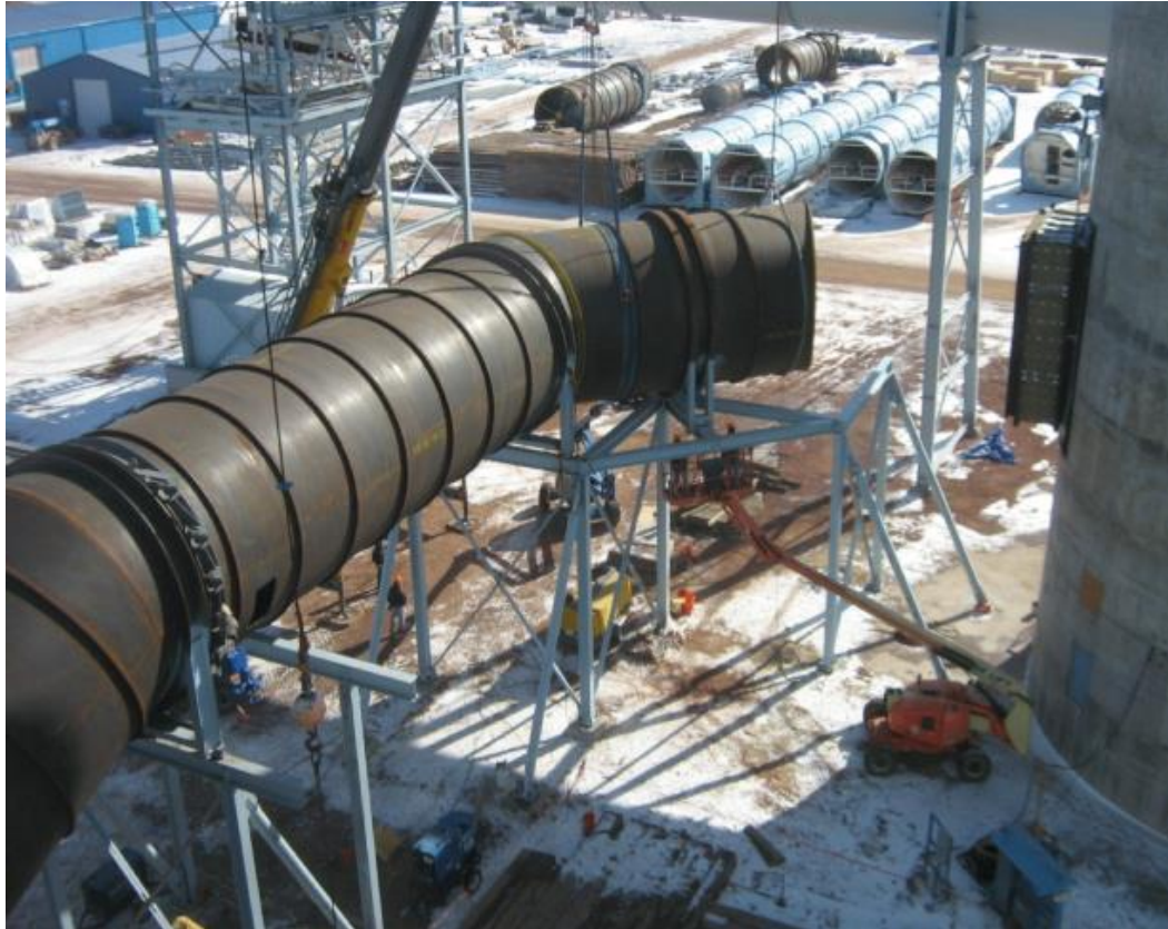
Photo During Construction
